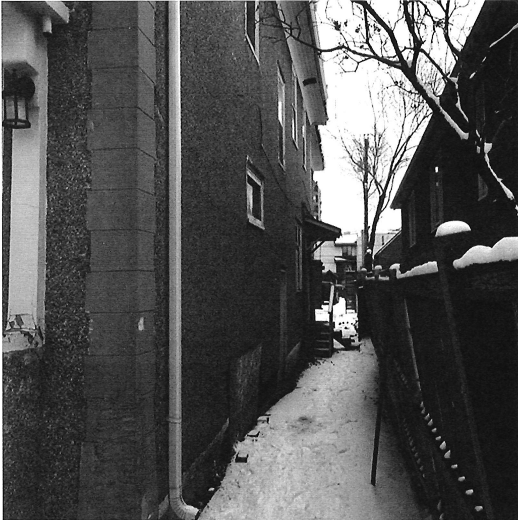
Rodd Apartments, 2016 – West Elevation
