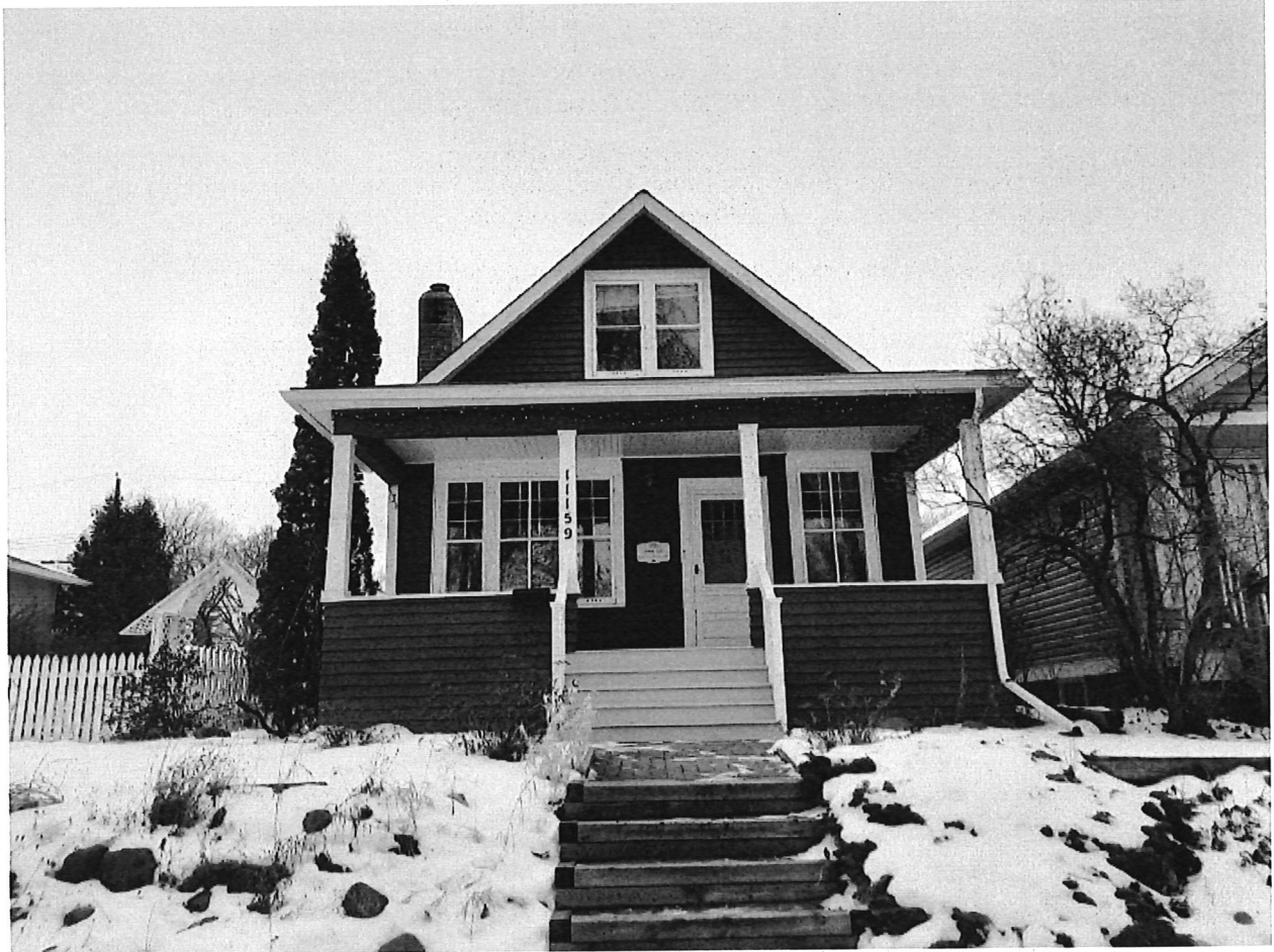
Photo #1 – Front (West) Elevation
