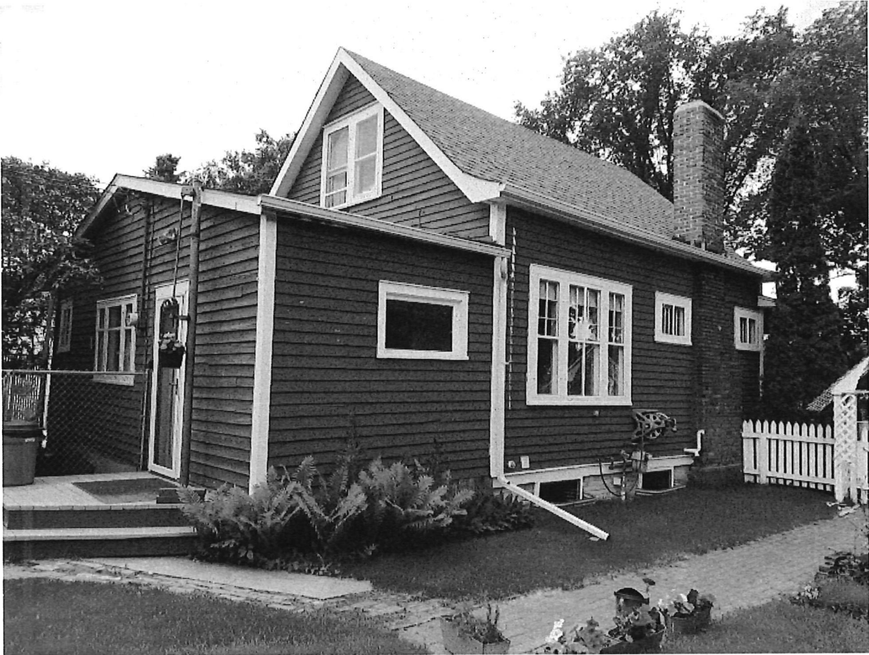
Photo #2 – Rear (West) and Side (North) Elevation
