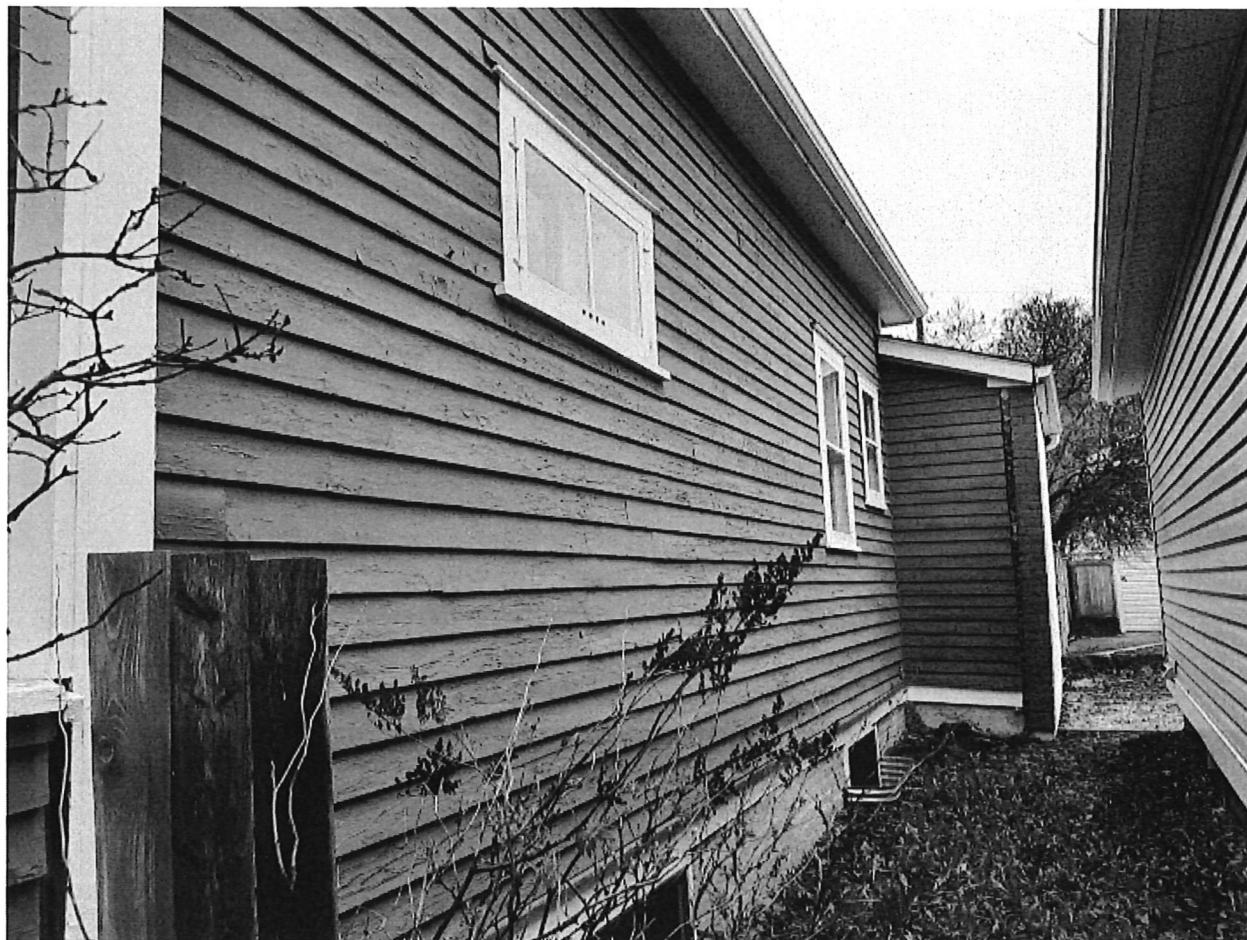
Photo #4 – Side (South) Elevation
